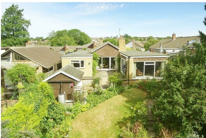
View of rear of house
